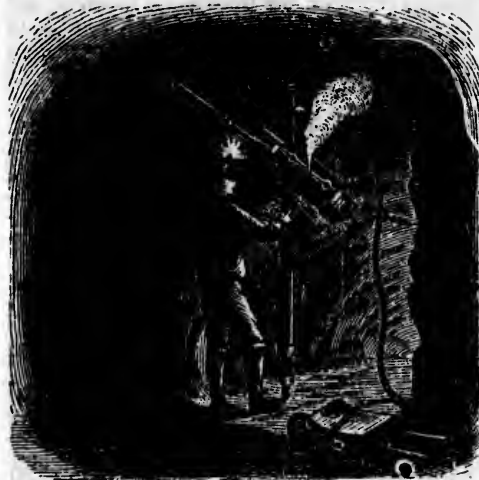
VIEW OF THE DRILL ATTACHED TO COLUMN, AS USED WITH COMPRESSED AIR OR STEAM, WHEN PRACTICABLE.
